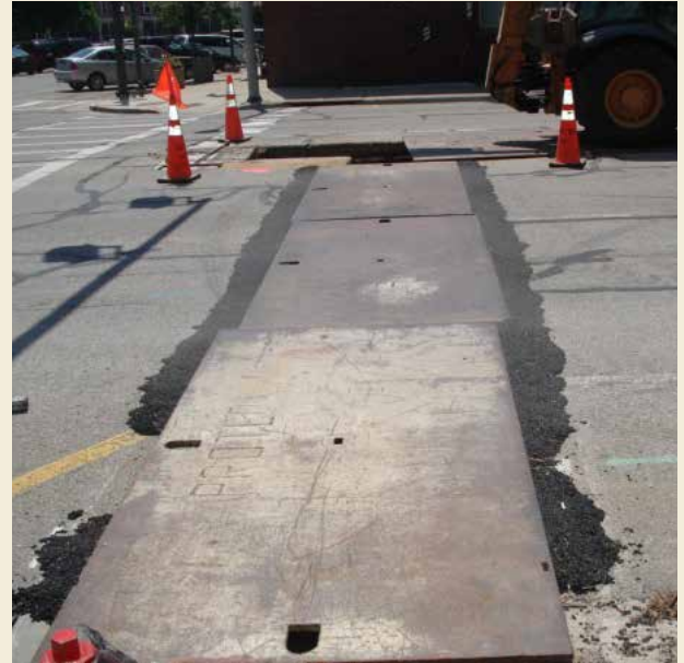
Steel Road Plates
