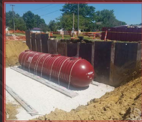
FUEL TANK INSTALL
